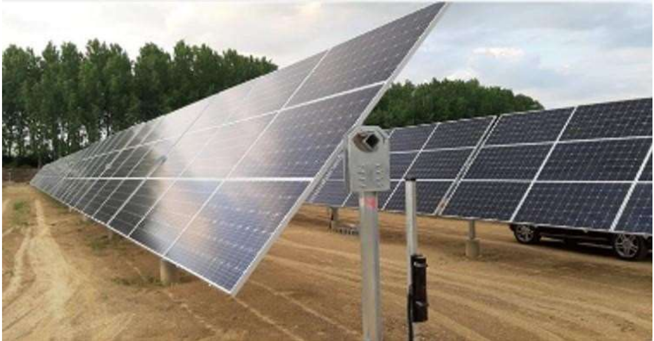
Figure 13: Tracking mechanism providing max 60° tilt angle to the north (i.e. about a fixed E-W axis)
