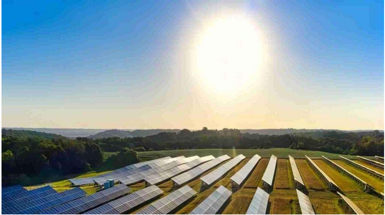
Figure 12: Typical Arrays oriented True North, with low angle setting sun in the
